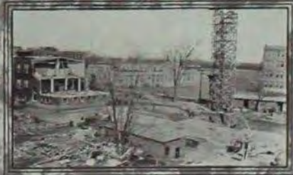
CONSTRUCTION STARTED ON MEC BUILDING
