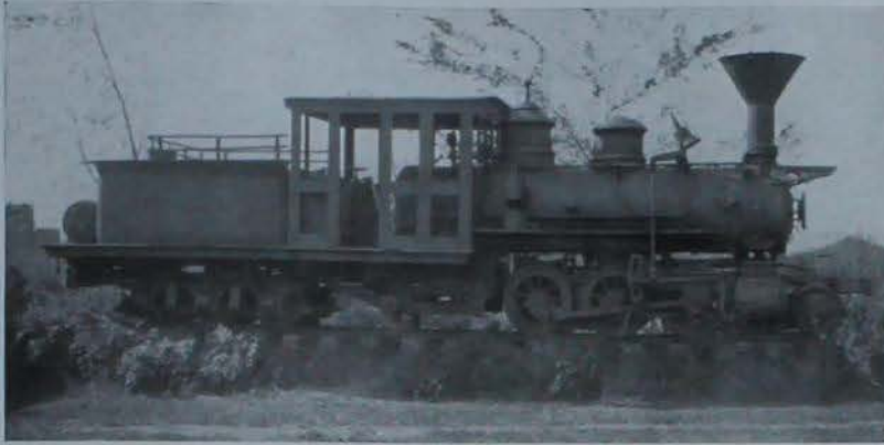
THE FIRST LOCOMOTIVE TO CROSS THE STATE OF IOWA
