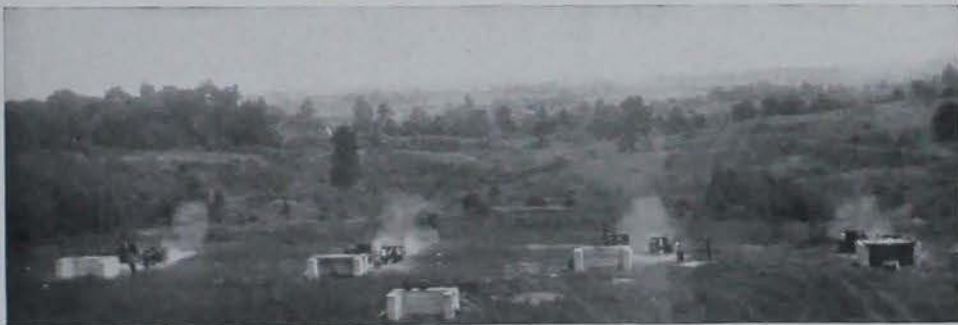
BATTERY IN ACTION AT CAMP KNOX
