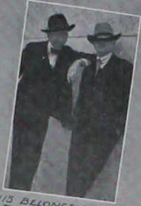
THIS BELONGS WITH THE AMES TANKS
