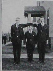
NO PLACE FOR THIS EXCEPT THE COMIC SECTION
