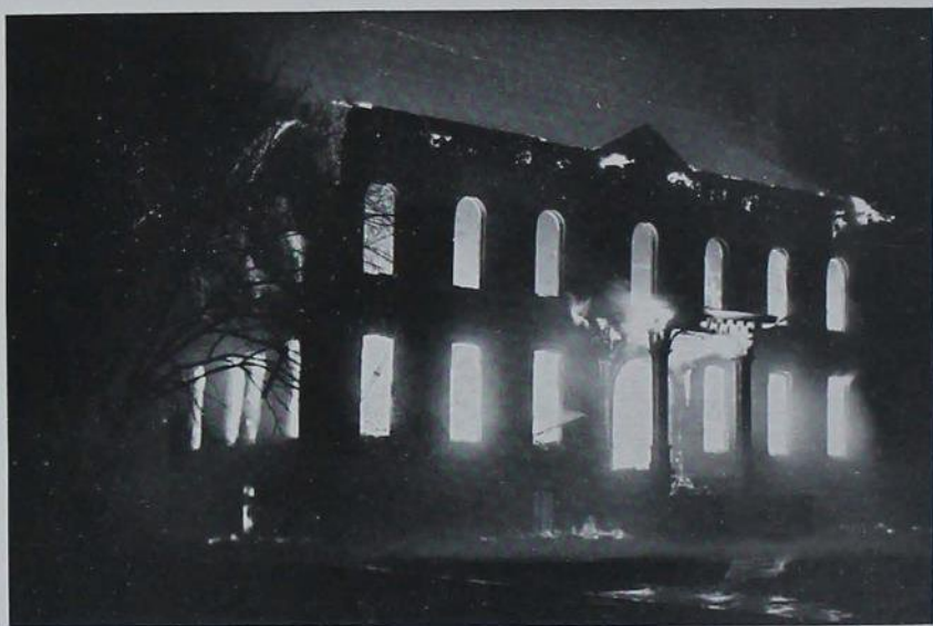
The South Wall Falls.
