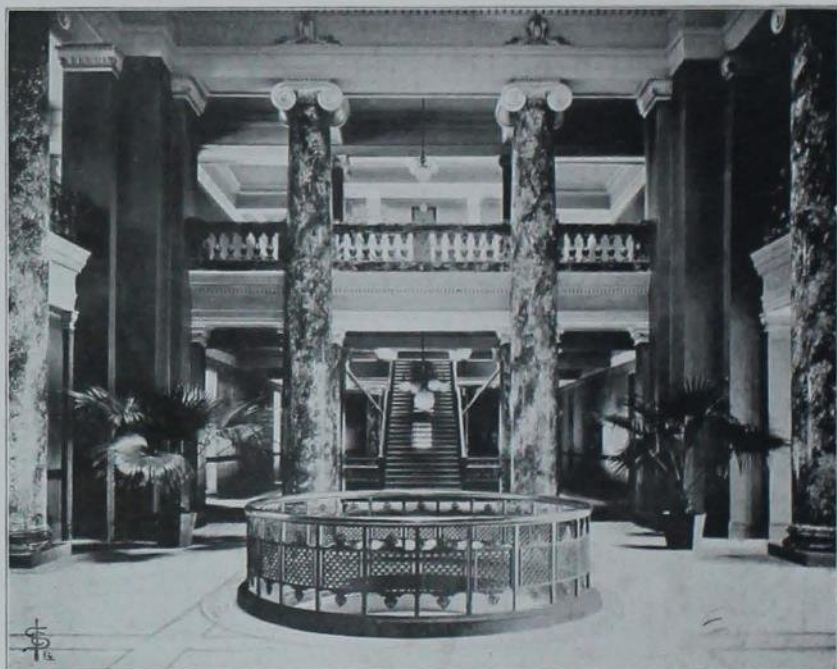
INSIDE OF NEW MAIN
