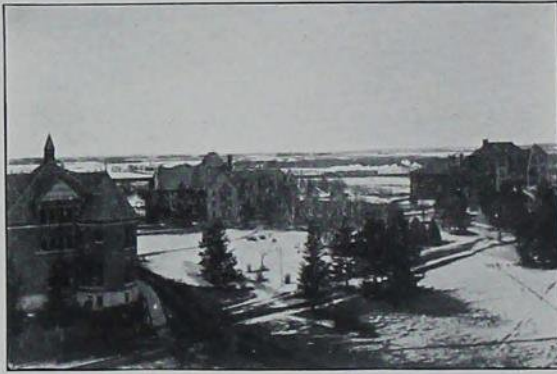
NORTHEAST FROM CENTRAL BUILDING—1905
