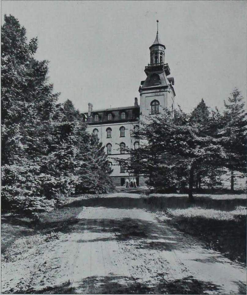
DRIVE NORTH FROM OFFICE.
