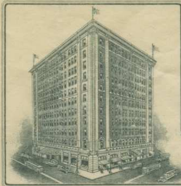
HOTEL BLACKHAWK 400 ROOMS 400 BATHS SERVIDOR SERVICE
